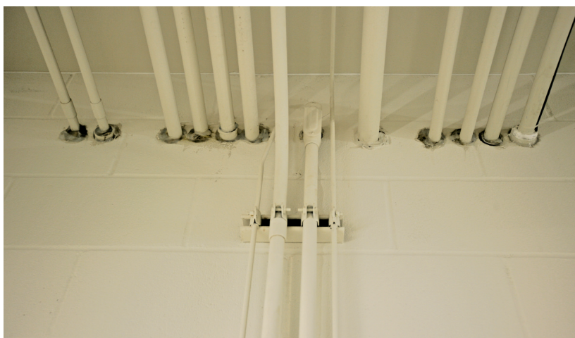
FIGURE 18. Caulking around Service Intrusions*
