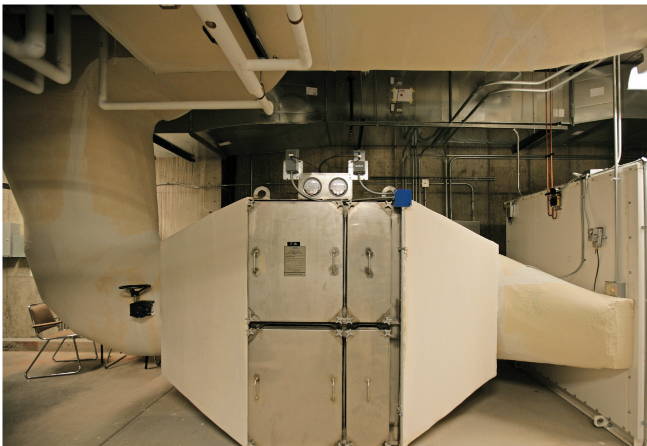
FIGURE 15. Bag-In, Bag-Out HEPA Filter System Attached to Air Handler*
